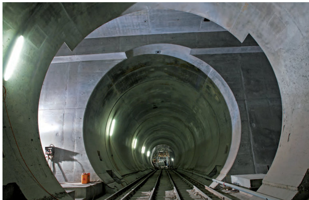
The recesses for the crossover tunnel doors are currently under construction.
