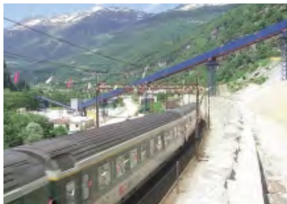
Around 2.2 million tonnes of spoil from the Faido section will be moved via a 5 km conveyor belt to fill an abandoned quarry at Cavienna, allowing the area to be restored
