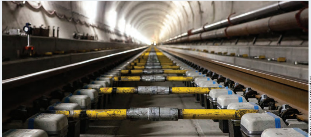
Right: Fit-out. The narrow-gauge construction railway is still in place as fitting out progresses in the Amsteg section.
