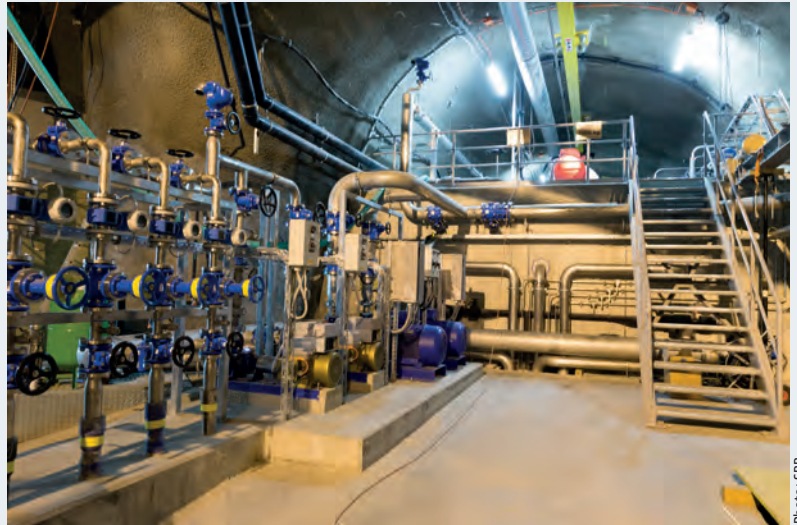
Machine room. Ventilation, drainage and pumping equipment is located in sealed rooms inside the tunnel.
