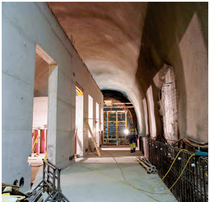
Construction of the railway equipment room is well advanced next to the traction power feed at Amsteg.
