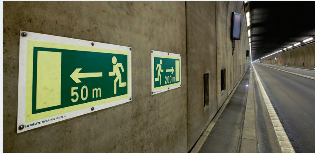
Photo: Federal Roads Office Fedro
