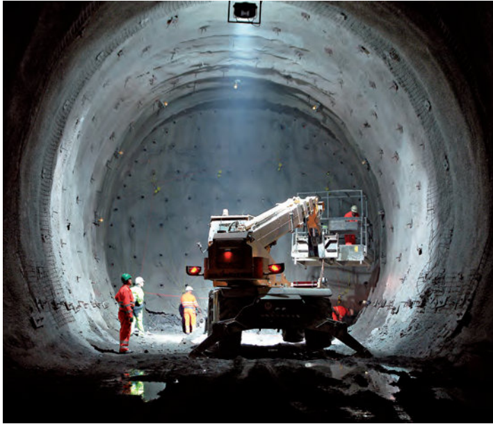
Work in progress at one of the faces at Sigirino in the centre of the Ceneri base tunnel.
