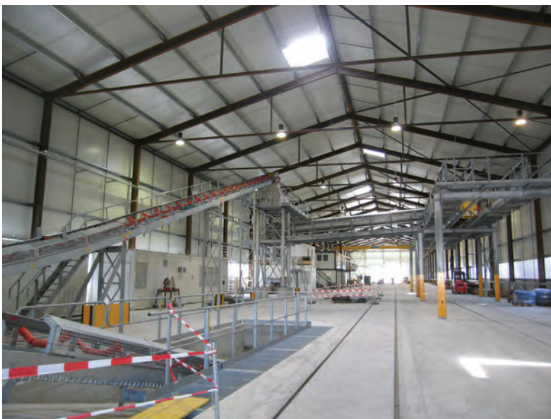
The concrete train spends two shifts in the tunnel. During the third shift it returns to the base at Erstfeld for a thorough clean before reloading. Facilities at Erstfeld include the cleaning and loading plant (left). About four or five days of material will be stocked on site to keep the train replenished.
