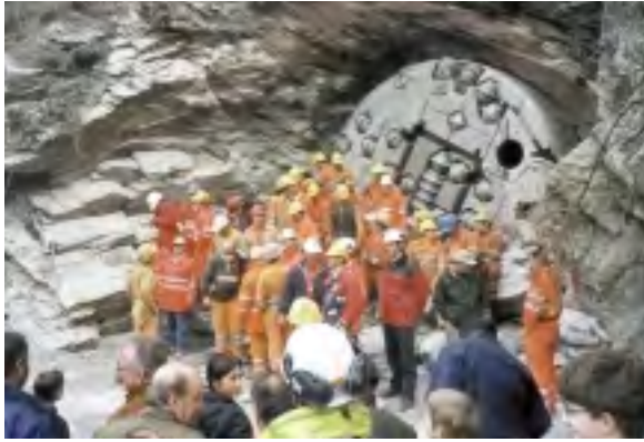
A ceremony was held at Bodio earlier this year (above) to mark the holing-through of a 3.2 km tunnel. Completed in nine months, this will carry spoil away from the southern worksite. The 6 km conveyor belt linking Bodio with a disposal area in the Blenio valley is now being installed (below right)
