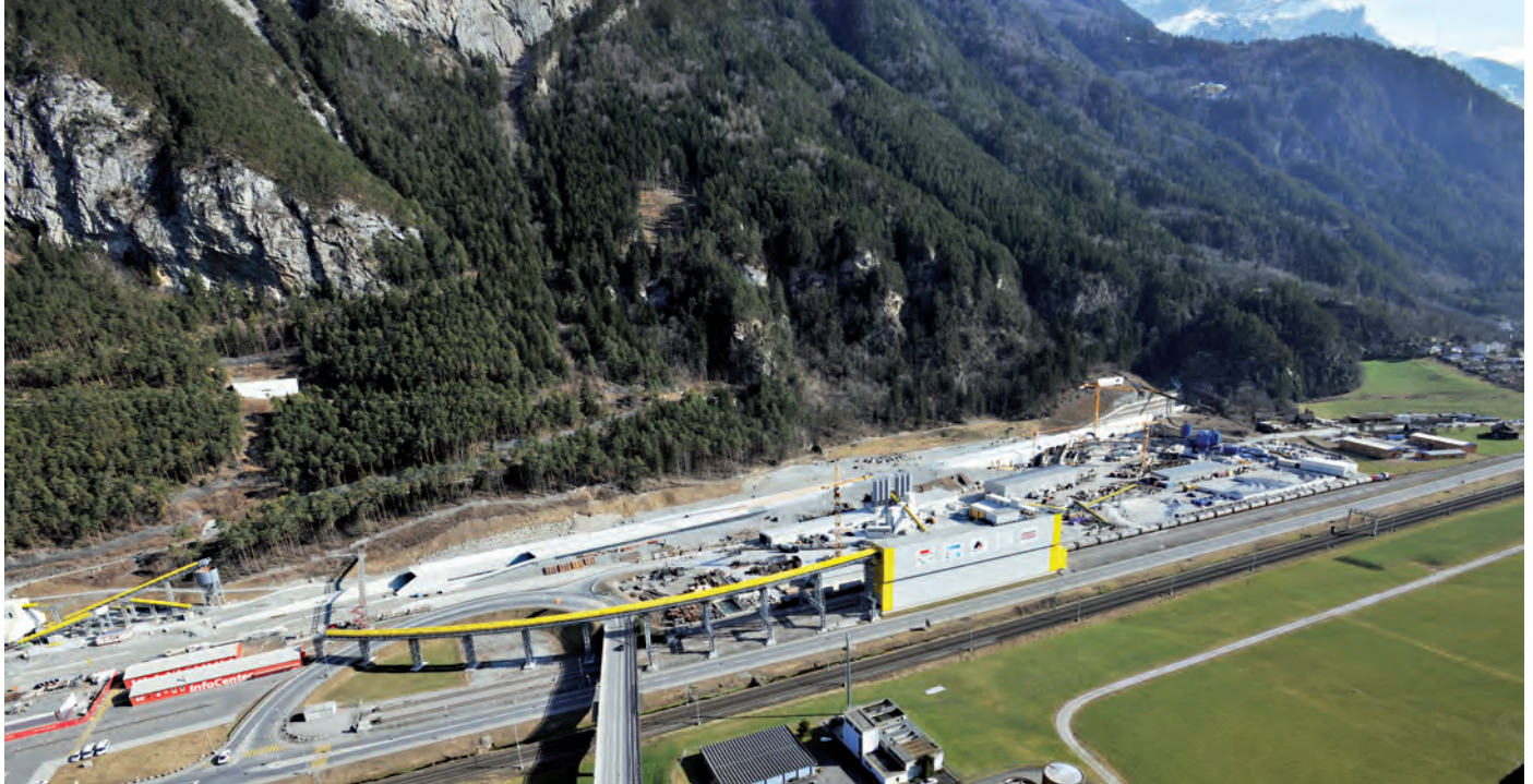
Aerial view of the Erstfeld cut-and-cover tunnel and the railway equipment building.
