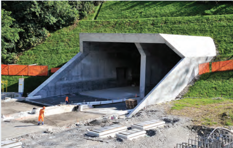
Going in. The northern portal of the Ceneri Base Tunnel at Vigana has been completed.
