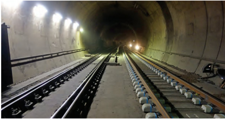
The LVT support blocks on one track in the Heitersberg tunnel (right) were renewed in 2014 using a series of short possessions.
