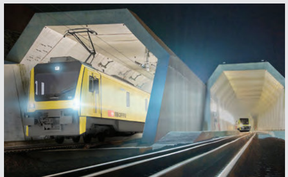
The dual-mode maintenance vehicles for the Gotthard Base Tunnel are being supplied by Harsco Rail.
