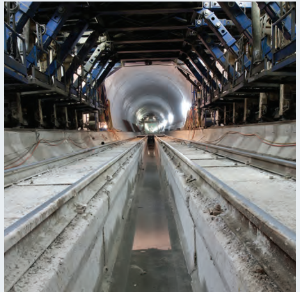
Right: Fit-out. The narrow-gauge construction railway is still in place as fitting out progresses in the Amsteg section.
