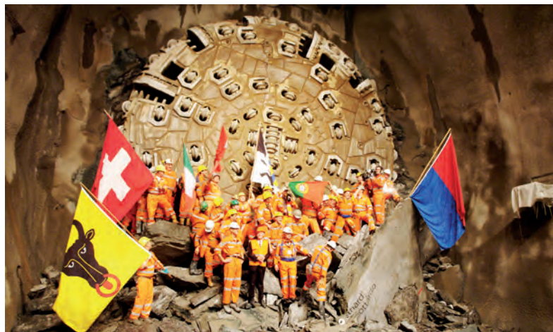
The breakthrough in the eastern bore was 30 km from the north portal and 2 500 m below Piz Vagira. Herrenknecht tunnel boring machine 'Sissi' had deviated just 10 mm from the vertical and 80 mm from the horizontal alignment.
