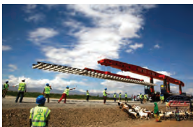
CCECC has begun tracklaying in Ethiopia on the new standard-gauge line under construction between Addis Ababa and Djibouti.
