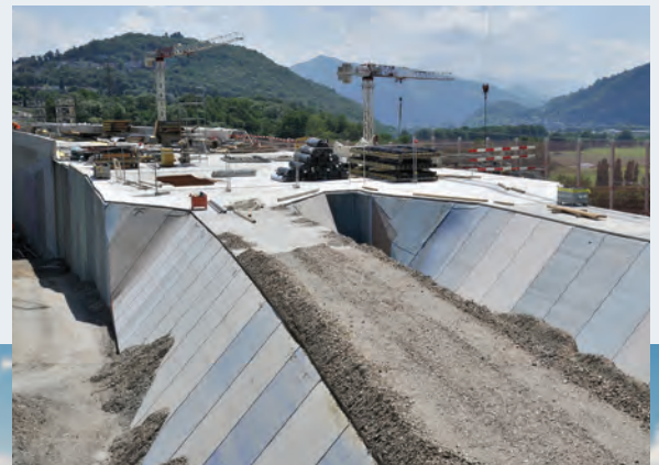
Coming out. Construction of the southern portal at Vezia was complicated by the presence of buildings very close to the alignment.
