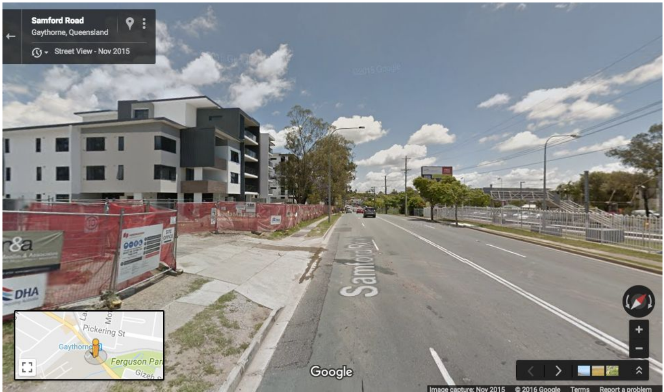
Figure 4: An example of what we are proposing across Brisbane. A Defence Housing Australia development at Gaythorne Station - five storeys, opposite railway station. Image: Google Maps.
