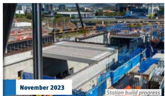
Station excavation progress
