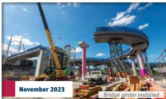
Bridge build progress
