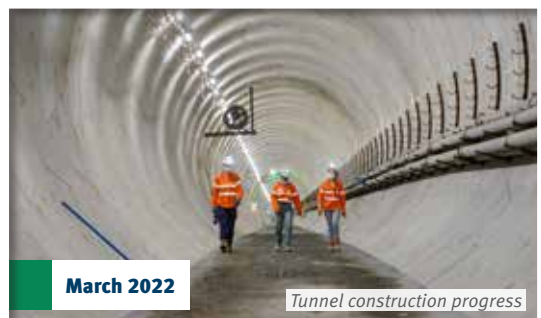
Construction of the tunnels
