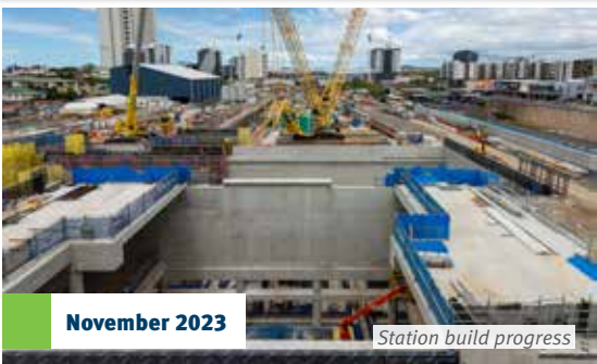
Station build progress
