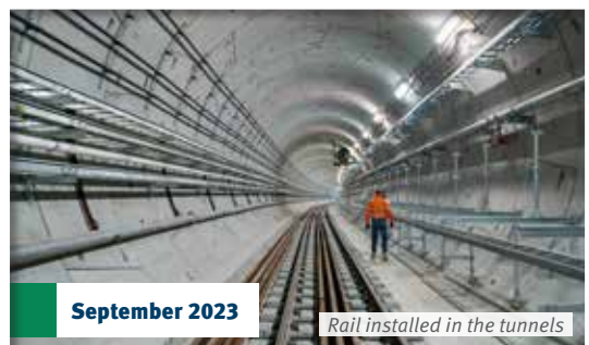
Tunnel construction progress
