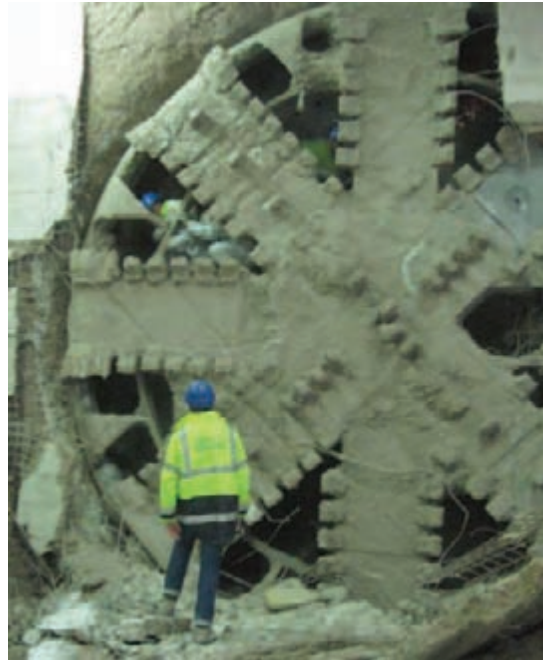
TBM breakthrough
