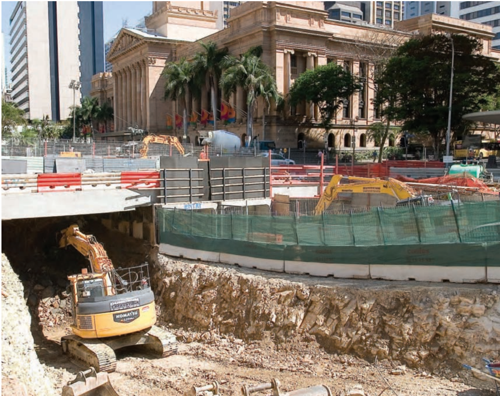
Above: Cut and cover construction
