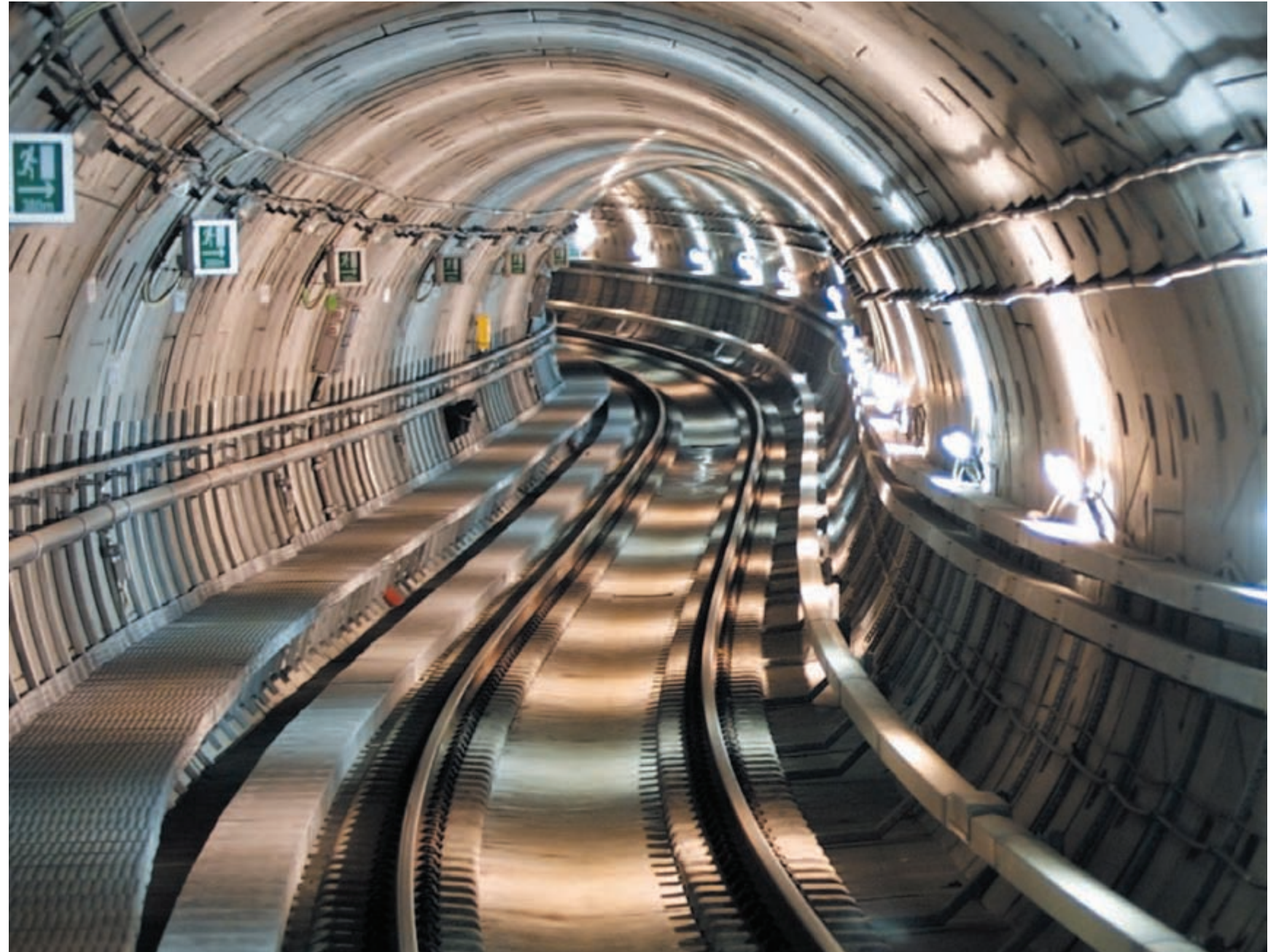
Commissioned tunnel infrastructure
