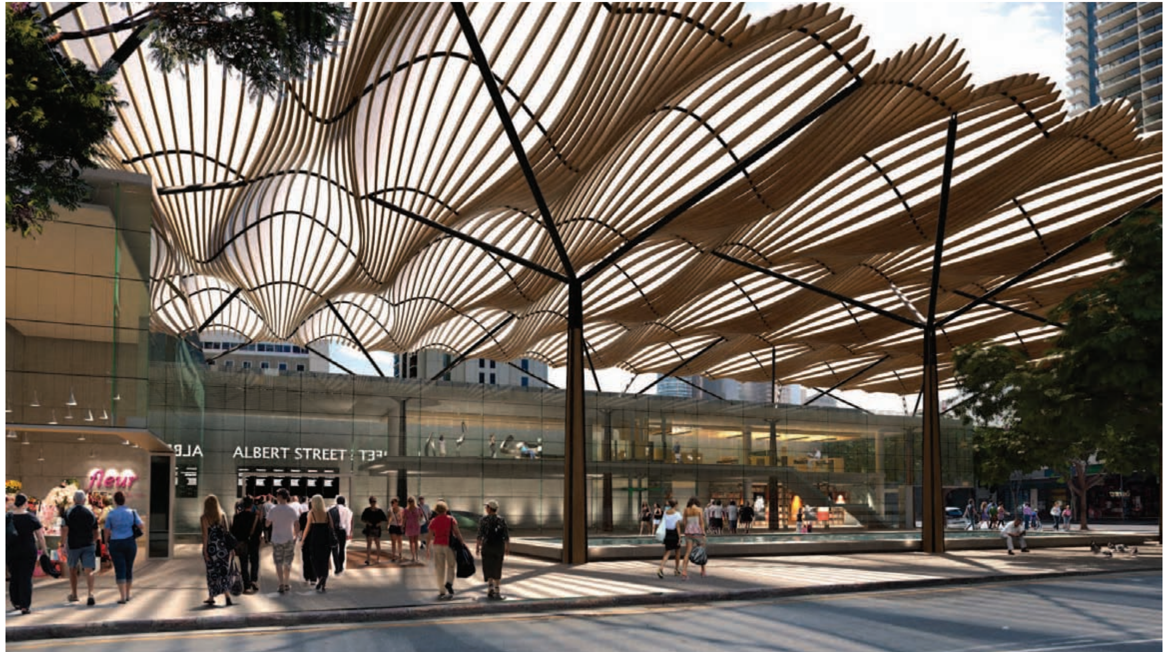
Albert Street Station – north entry at corner of Mary and Albert Streets
