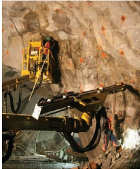
Rock bolt installation
