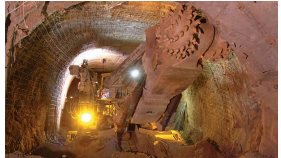
Above left: Geotechnical investigations Top: Roadheader construction Left: Tunnel boring machine (TBM)
