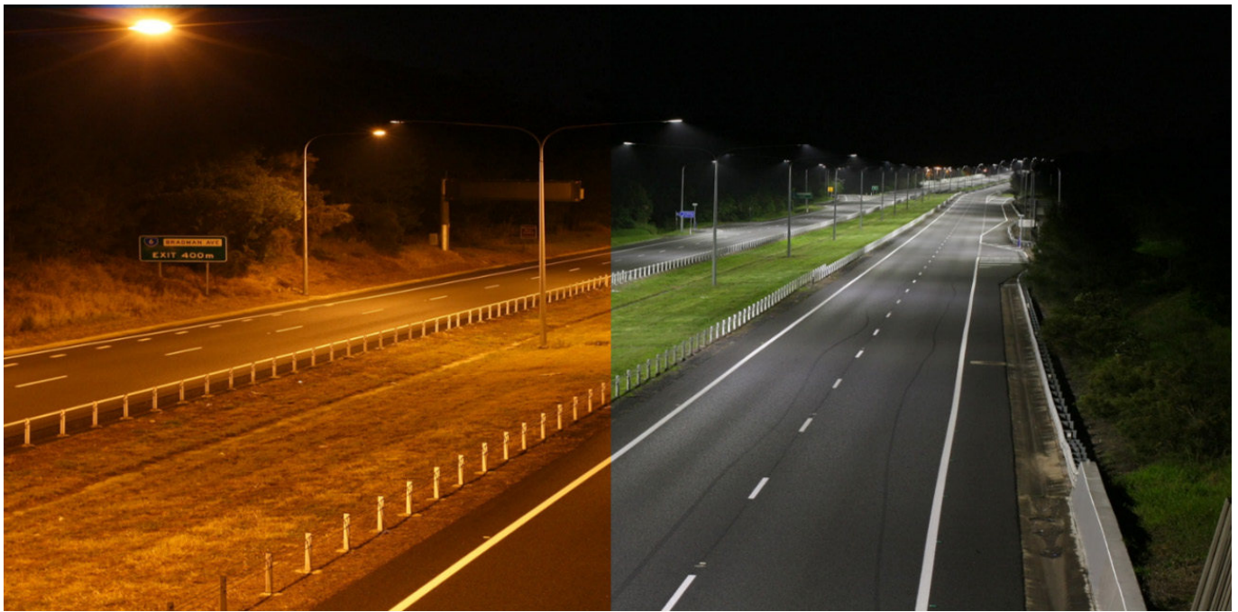
Before and after LED installation on the Sunshine Motorway showing the improved visibility for motorists.
