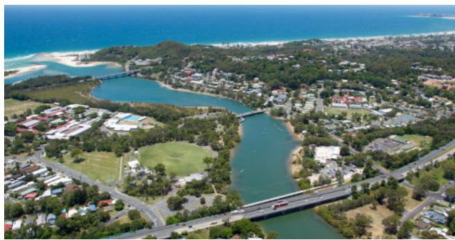
Pacific Motorway Currumbin Creek Bridge.
