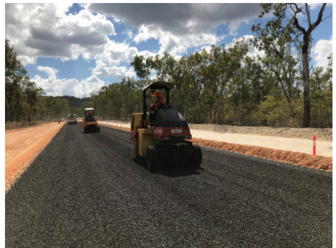
Sealing works at Ten Mile Creek
