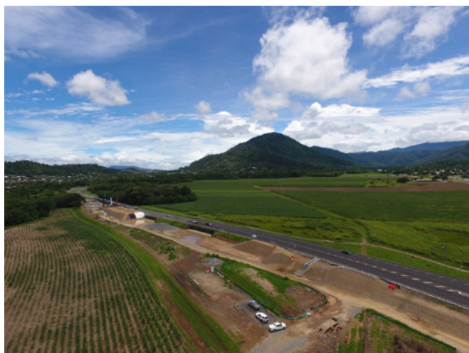
Duplication of Bill Fulton Bridge was one of the highest priority infrastructure projects in Cairns for many years.
