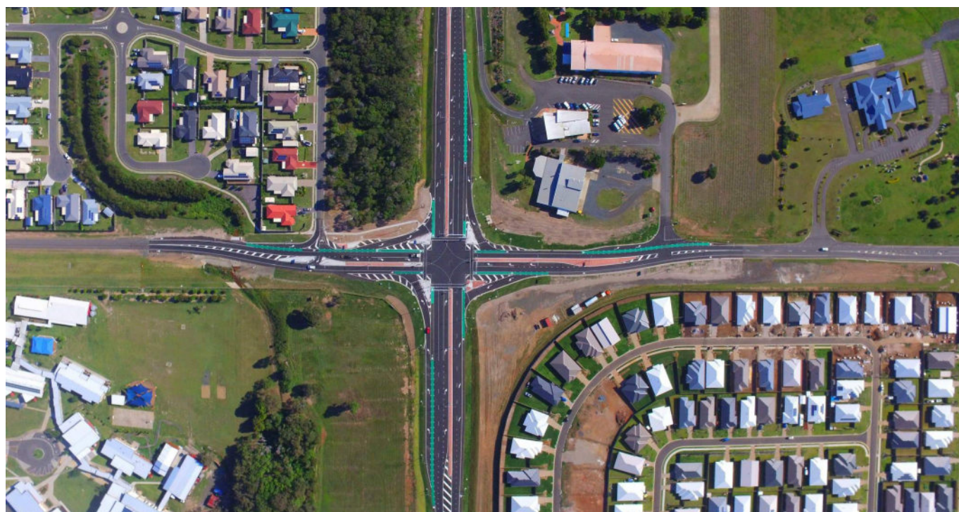
Aerial photo of upgraded Urraween Road intersection.
