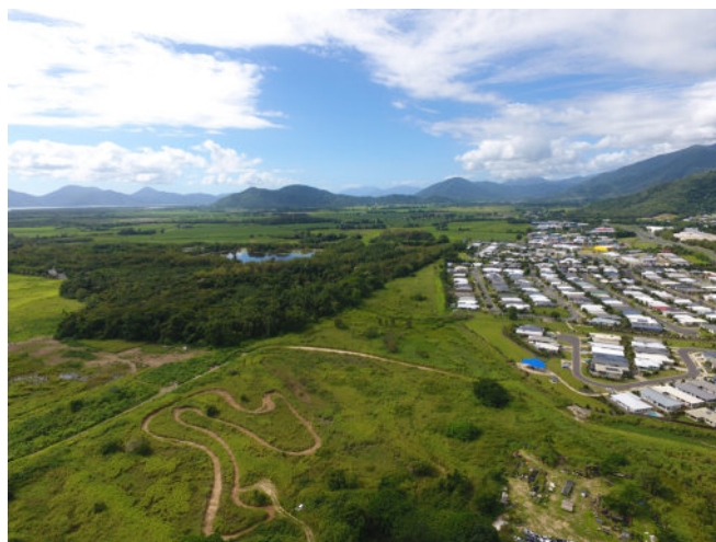
Looking south along the alignment of the future Smithfield Bypass Road, which passes around Cattana Wetlands.
