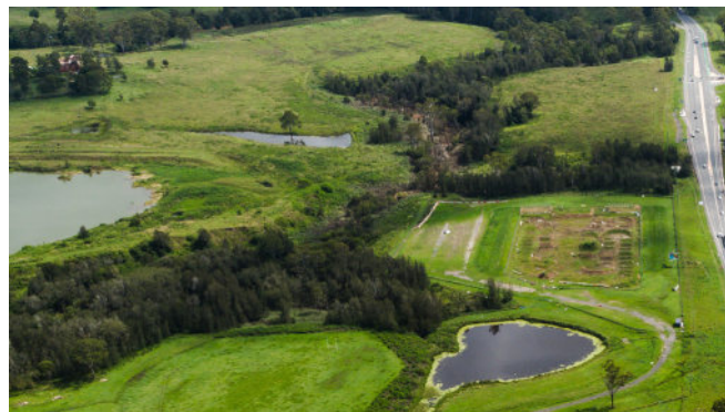
Mount Lindesay Highway – Jimboomba (Johanna Street to Camp Cable Road Intersection, looking north).
