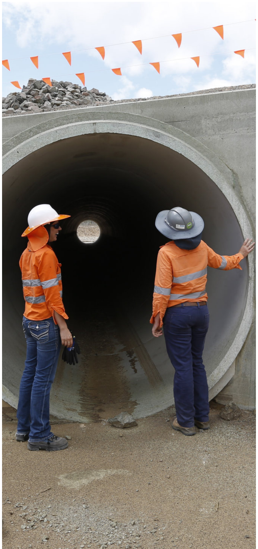
TMR staff inspecting construction
