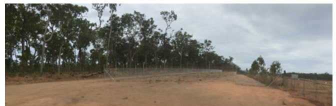
Clearing and fencing preparation works for the Mapoon Airstrip upgrade, July 2017.
