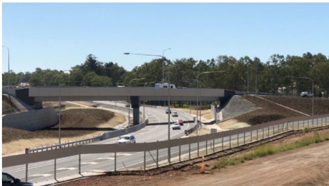
Bruce Highway Upgrade Program Tinana overpass completed in late 2017.
