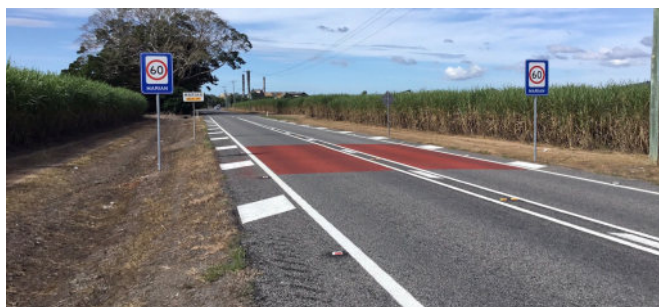
Township Entry Treatment installed at Marian on Eungella Road in Mackay.
