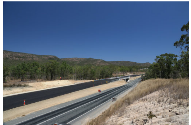
Peak Downs Highway Timber Bridges replacement project (Fiery Creek).
