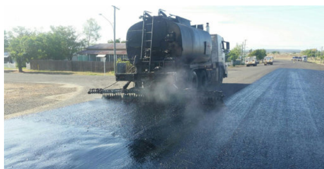
Rehabilitation work on Flinders Highway through Hughenden
