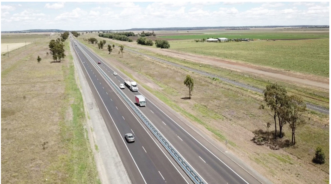
Opposing westbound and eastbound overtaking lanes, as part of the Oakey to Dalby Overtaking Lanes project.
