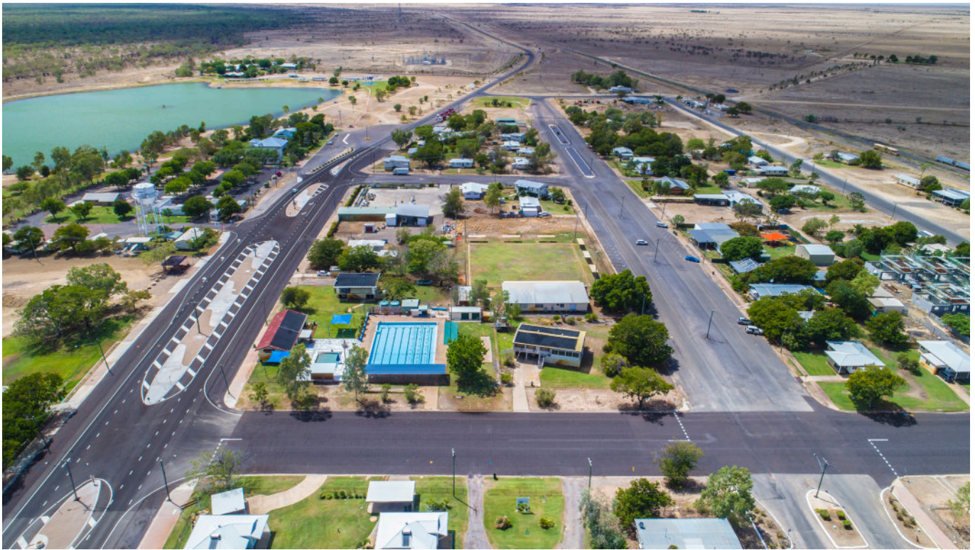
Completed works to Goldring Street, Richmond.
