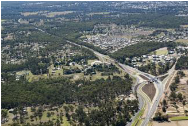
Looking north over the Tinana interchange on the Bruce Highway. Image provided courtesy of Georgiou Group.
